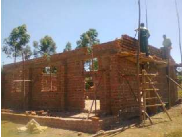
Bricklaying of the classroom
