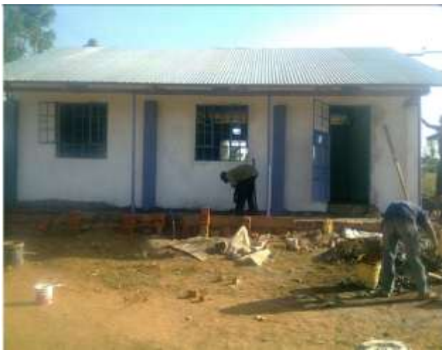
Painting the plastered exterior
