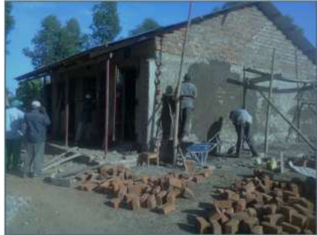
plastering over the brickwork
