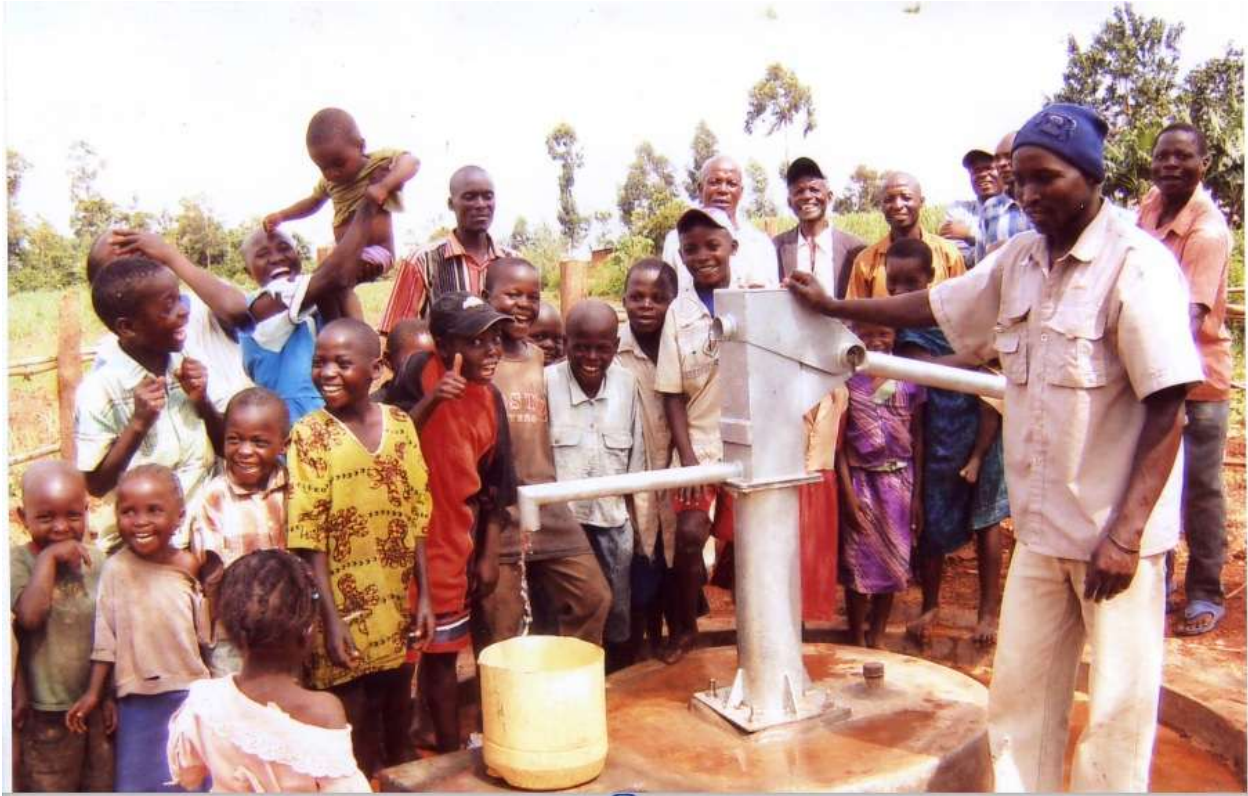
A new community well serves 500 people with clean water. This was a well installed by SFA at Sacred Shrine community, in Kakamba, Kenya.
